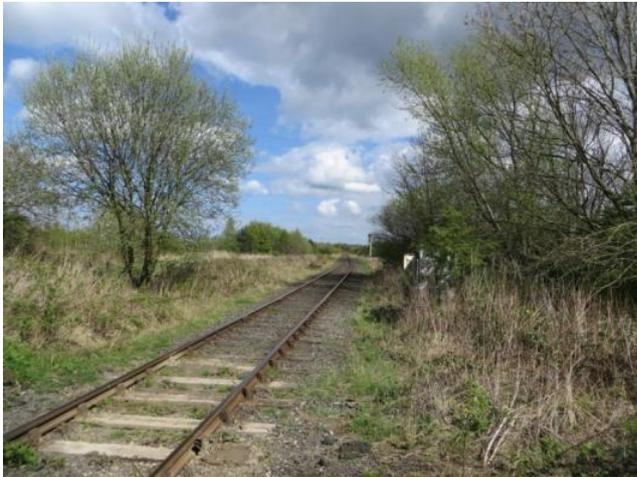
Figure 4: Looking east along the Harworth Estates' route from Linton Lane foot crossing. A good width is available between the railway land boundary fences for future double tracking. Taken on 6<sup>th</sup> May 2014.
